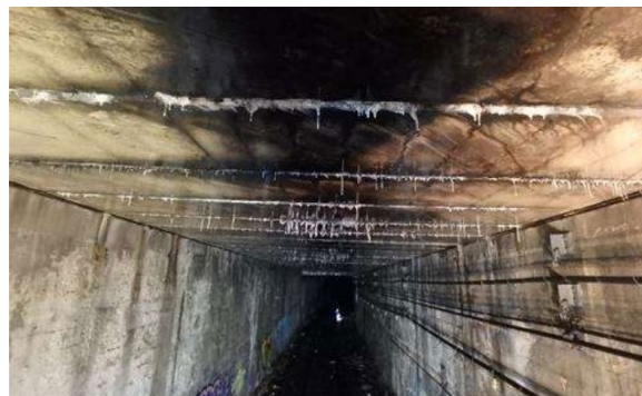
North Section of the Tunnel
