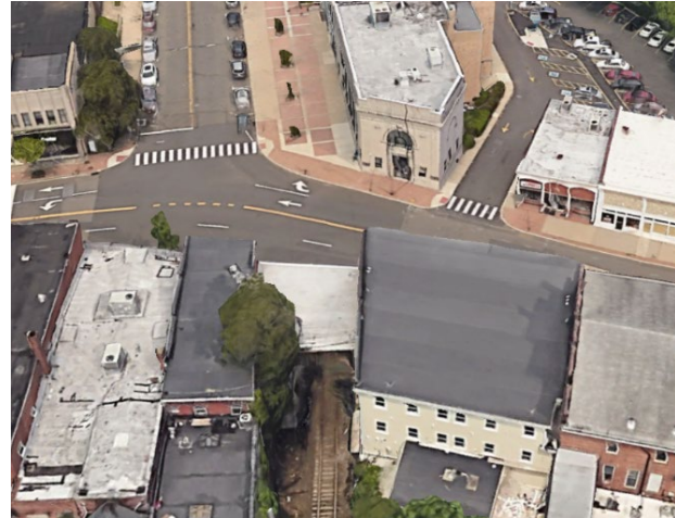
Wall St Tunnel – South Portal
