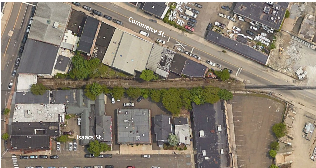
Figure 8: Isaacs Street Site (source: Google Earth)
