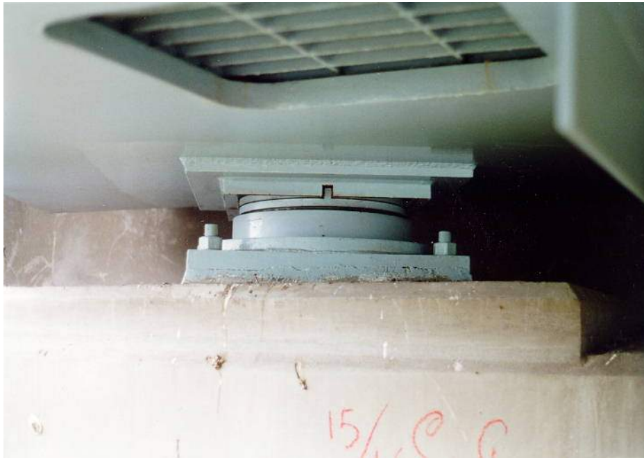
Figure 6.2.1o – Center Guided Pot Bearing
