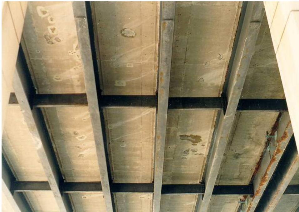
Figure 6.2.7a – Typical Rolled Multi-Stringer Superstructure with Ends of Partial Length Welded Cover Plates Visible.
