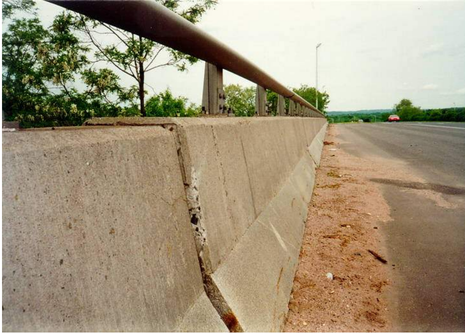
Figure 6.1.5b –Sloped Granite Curb on Concrete Parapet.
