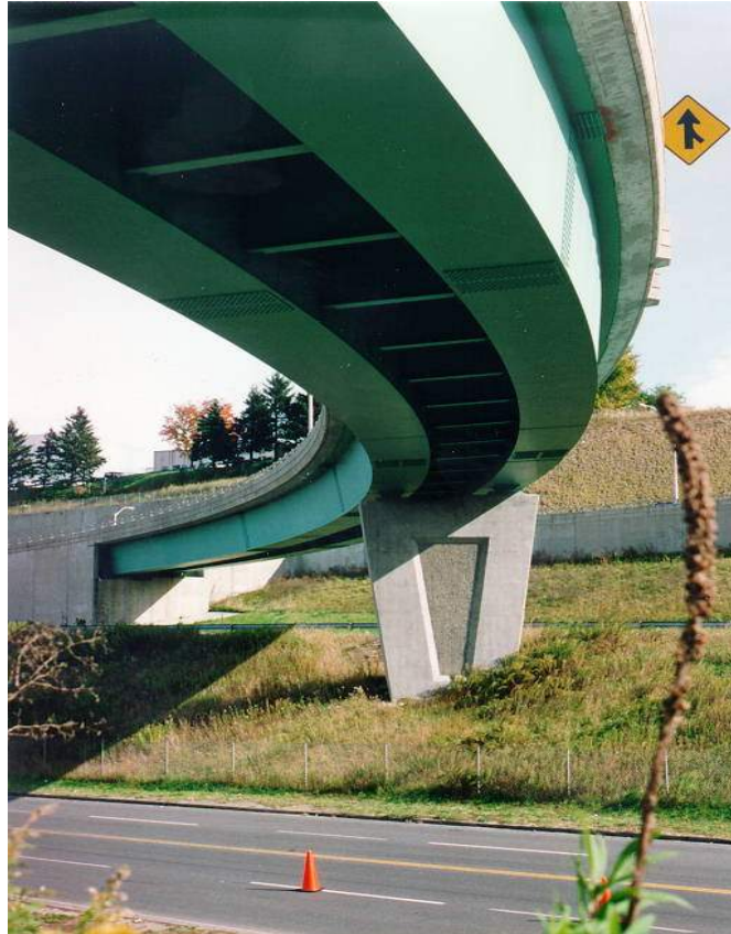
Figure 6.2.9a – Curved Steel Box Girder Bridge.
