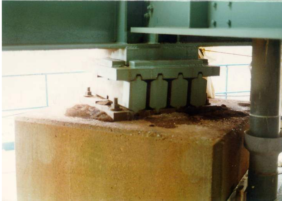
Figure 6.2.11 – Nested Rocker Bearing Used for Very Large Spans.
