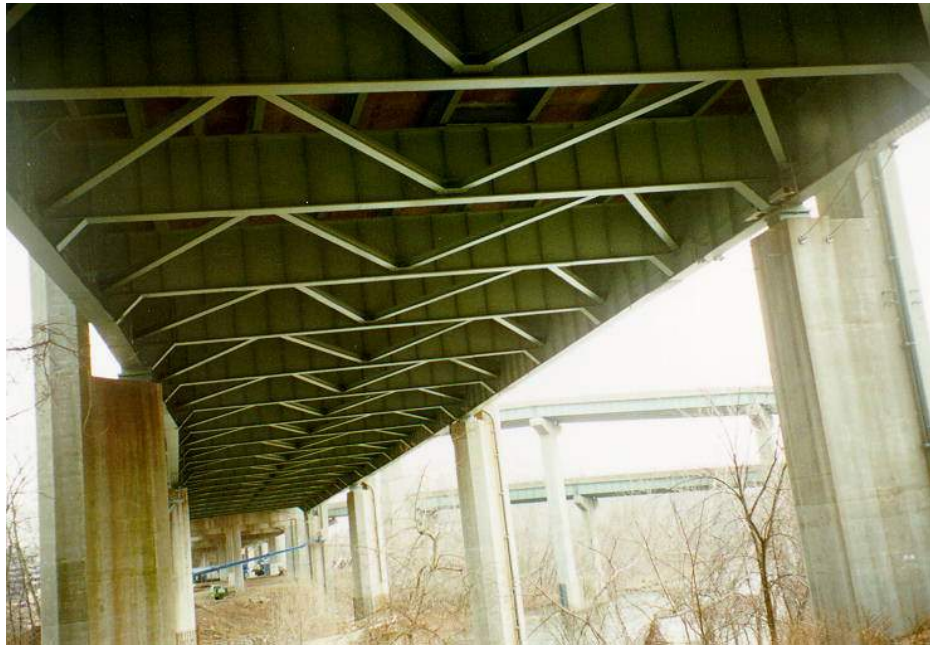
Figure 6.2.8a – Large Girder-Floorbeam-Stringer Bridge.
