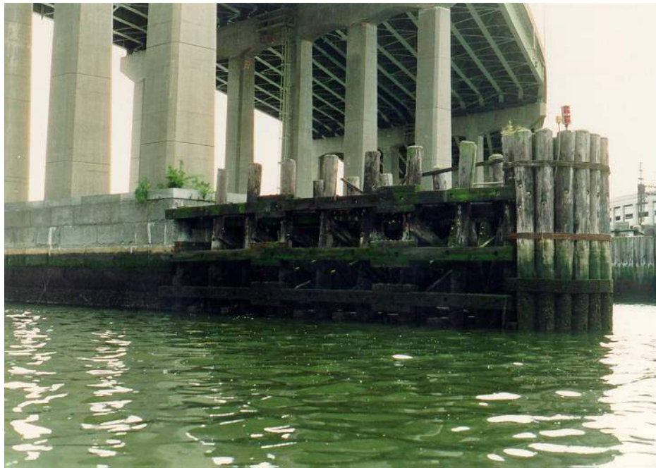
Figure 6.4.1a – Timber Fender System with Navigation Lights.
