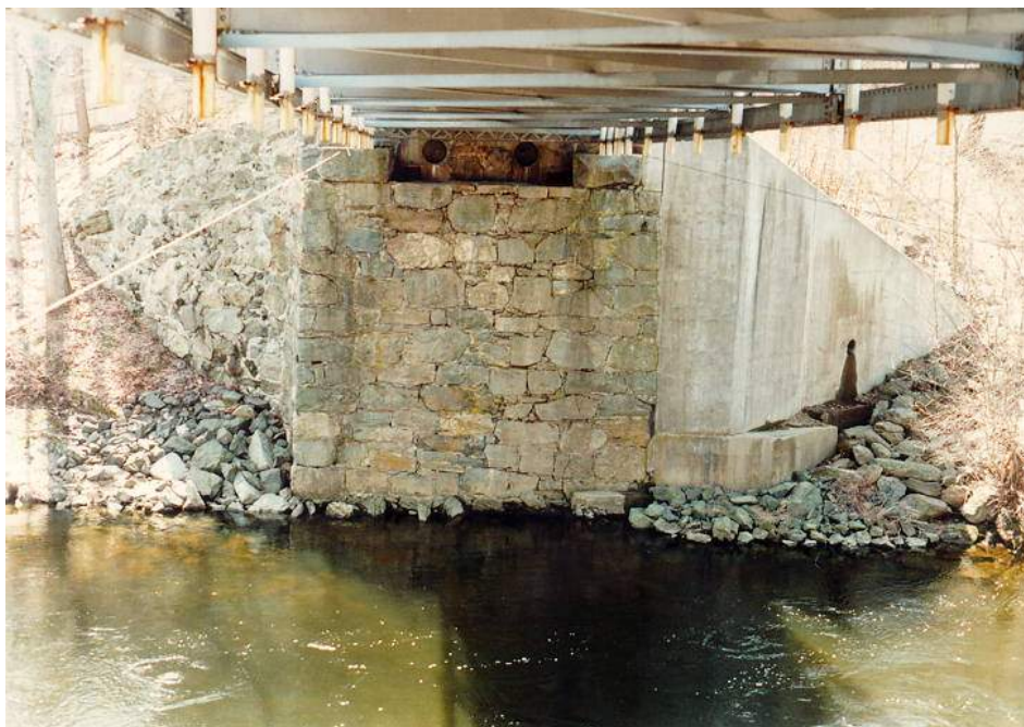
Figure 6.3.2a Tall Stone Masonry Bridge Abutment with Newer
