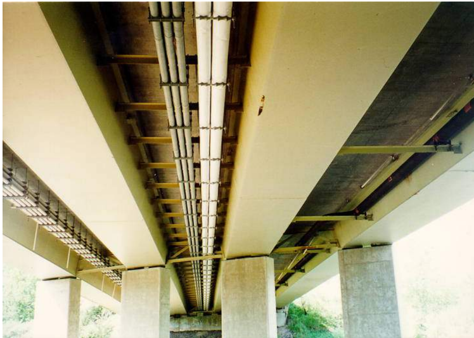
Figure 6.1.11a – Typical Under-Bridge Utility Installation
