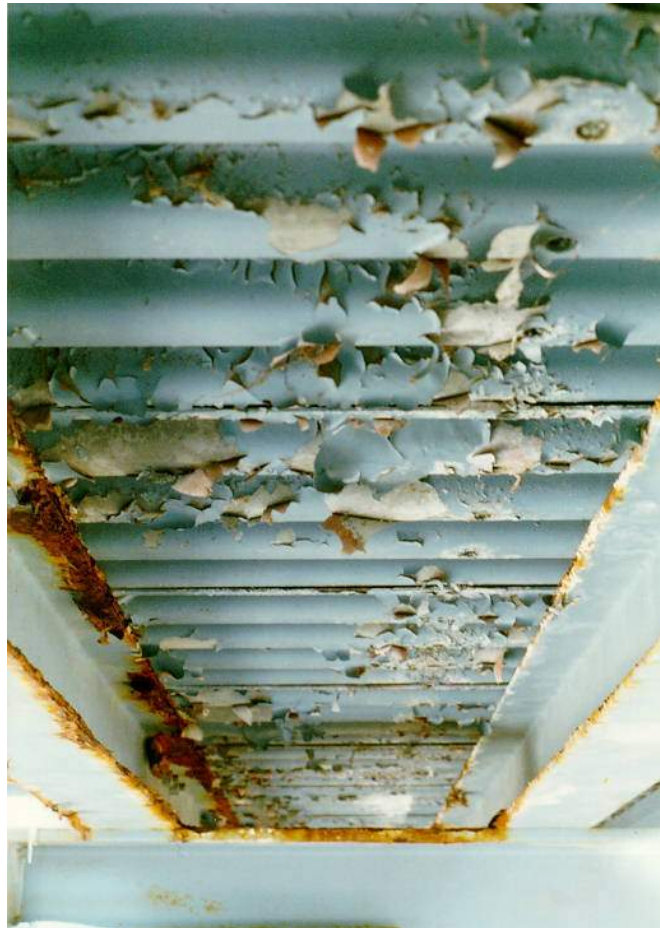
Figure 6.1.3a – Underside of Asphalt Filled Metal Deck Pans.
