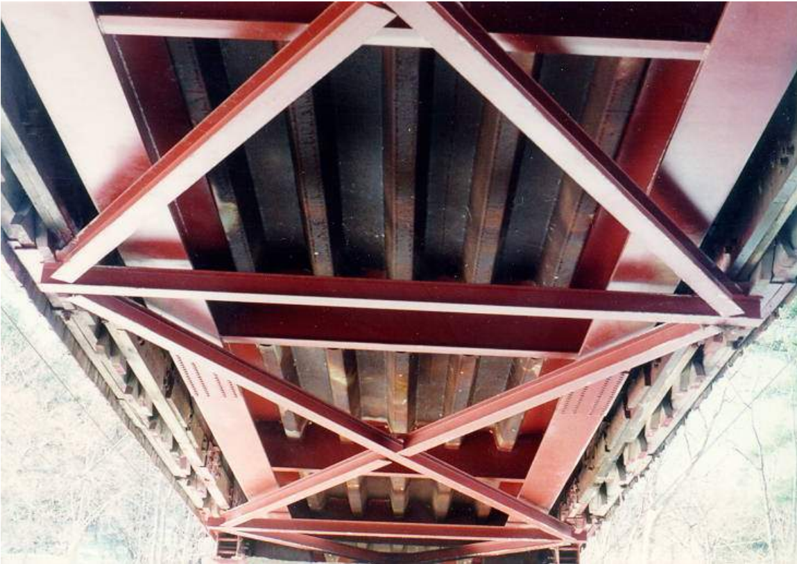
Figure 6.1.3b – Underside of Orthotropic Steel Plate Deck
