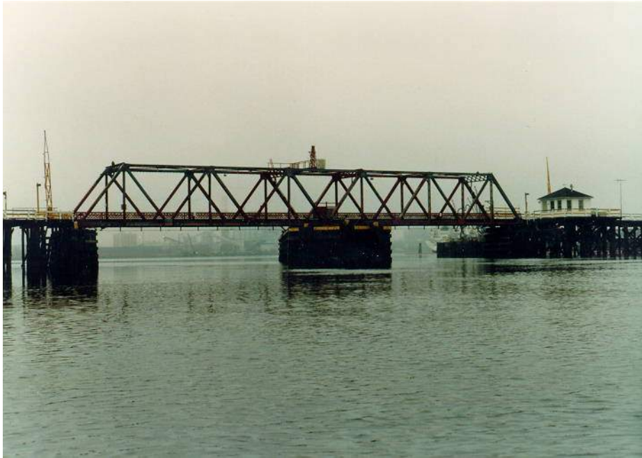
Figure 6.2.11a – Swing Span Truss Bridge.
