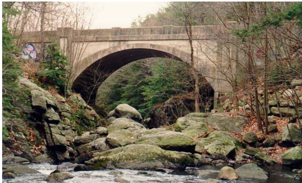
Figure 6.2.4a – A Closed Spandrel Reinforced Concrete Arch Bridge.
