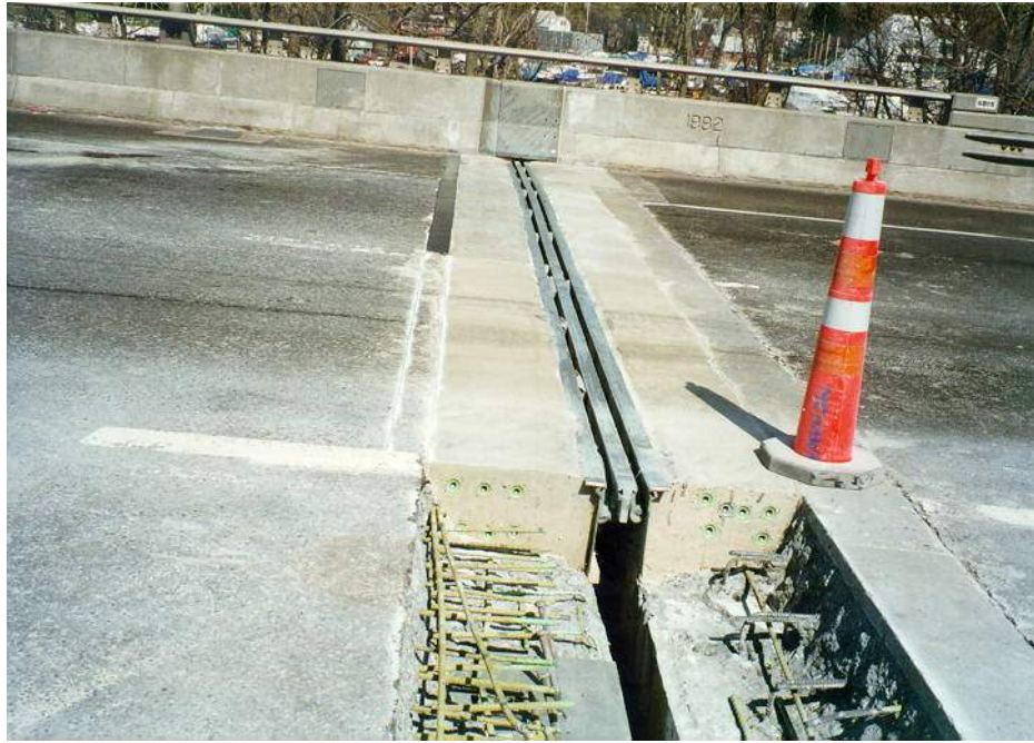
Figure 6.1.2c – Modular Type Expansion Joint.
