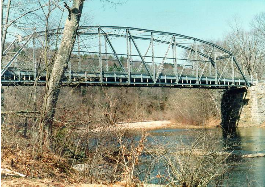
Figure 6.2.10a – Historic Steel Through Truss Bridge.
