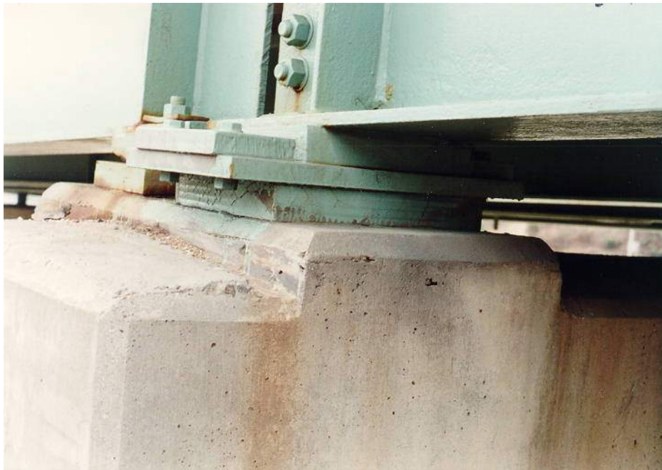
Figure 6.2.1k – Retrofit Detail. Elastomeric Bearing Installed to Replace Bronze Sliding Plate Bearing.
