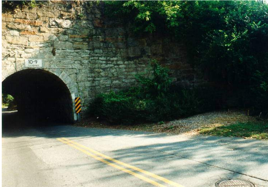
Figure 6.2.13b – Stone Masonry Arch Viaduct
