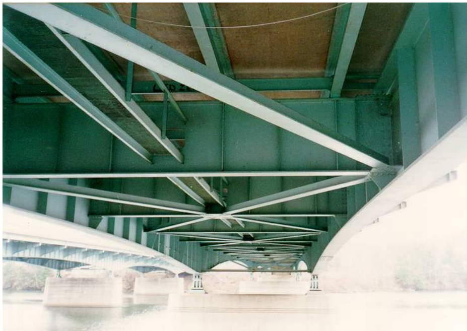
Figure 6.2.8b – Typical Framing on a Girder-Floorbeam-Stringer Superstructure.
