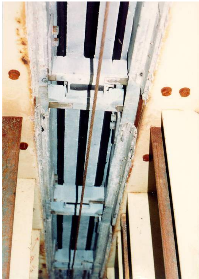
Figure 6.1.12d – Underside of Modular Joint.
