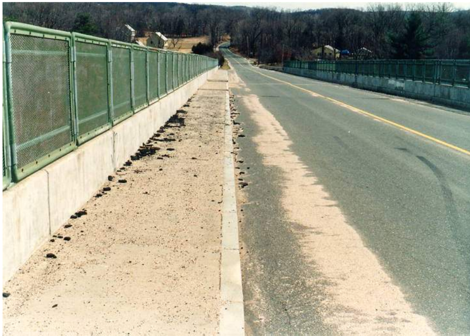
Figure 6.1.9b – Pedestrian Fence atop Concrete Parapet.
