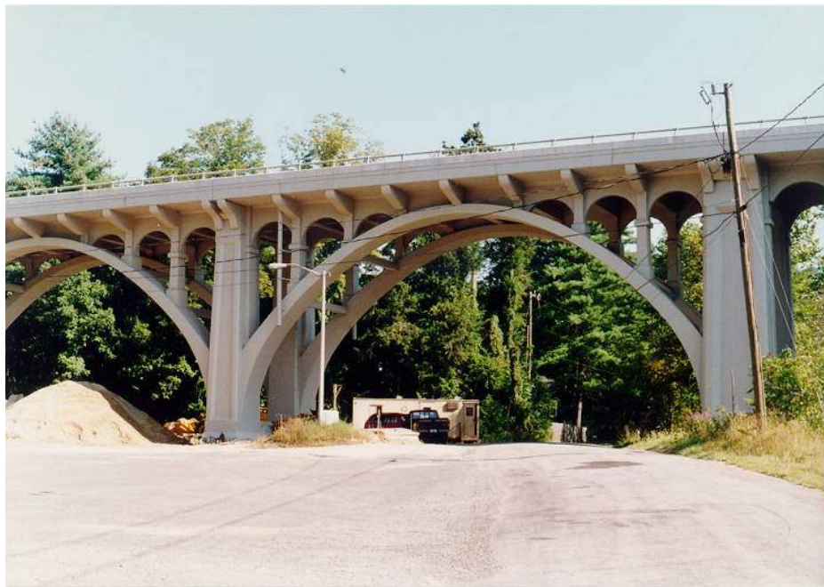
Figure 6.2.5a – Open Spandrel Concrete Arch Bridge.
