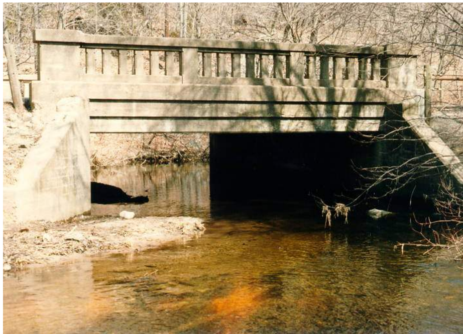
Figure 6.2.2a – Typical Concrete Slab Bridge.
